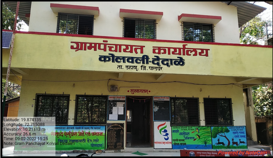
GRAM PANCHAYAT OFFICE, KOLAVALI AND DEDAHE
