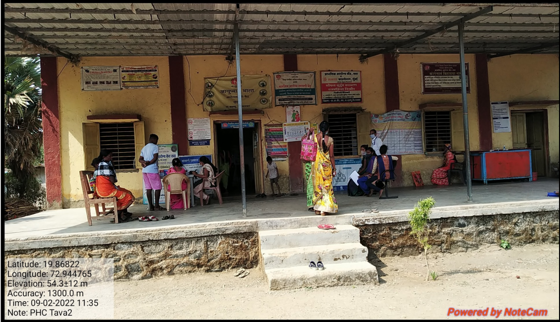
PRIMARY HEALTH CENTRE, VILLAGE TAWA
