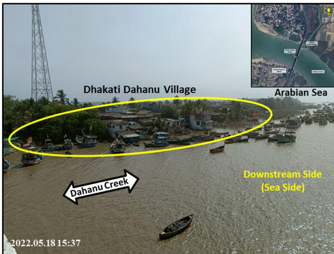
Photo 5 : View of Downstream of Dahanu Creek from Dahanu Road Bridge (During High Tide)
