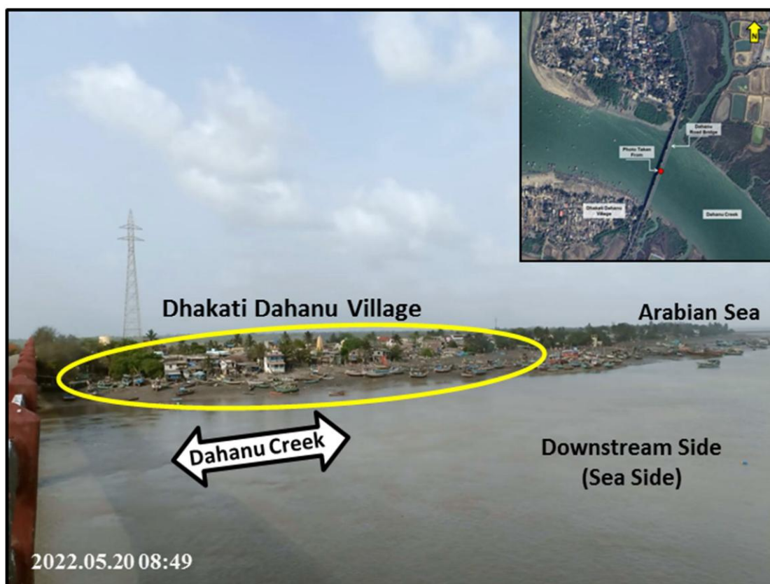
Photo 7 : View of Downstream of Dahanu Creek from Dahanu Road Bridge (During Low Tide)
