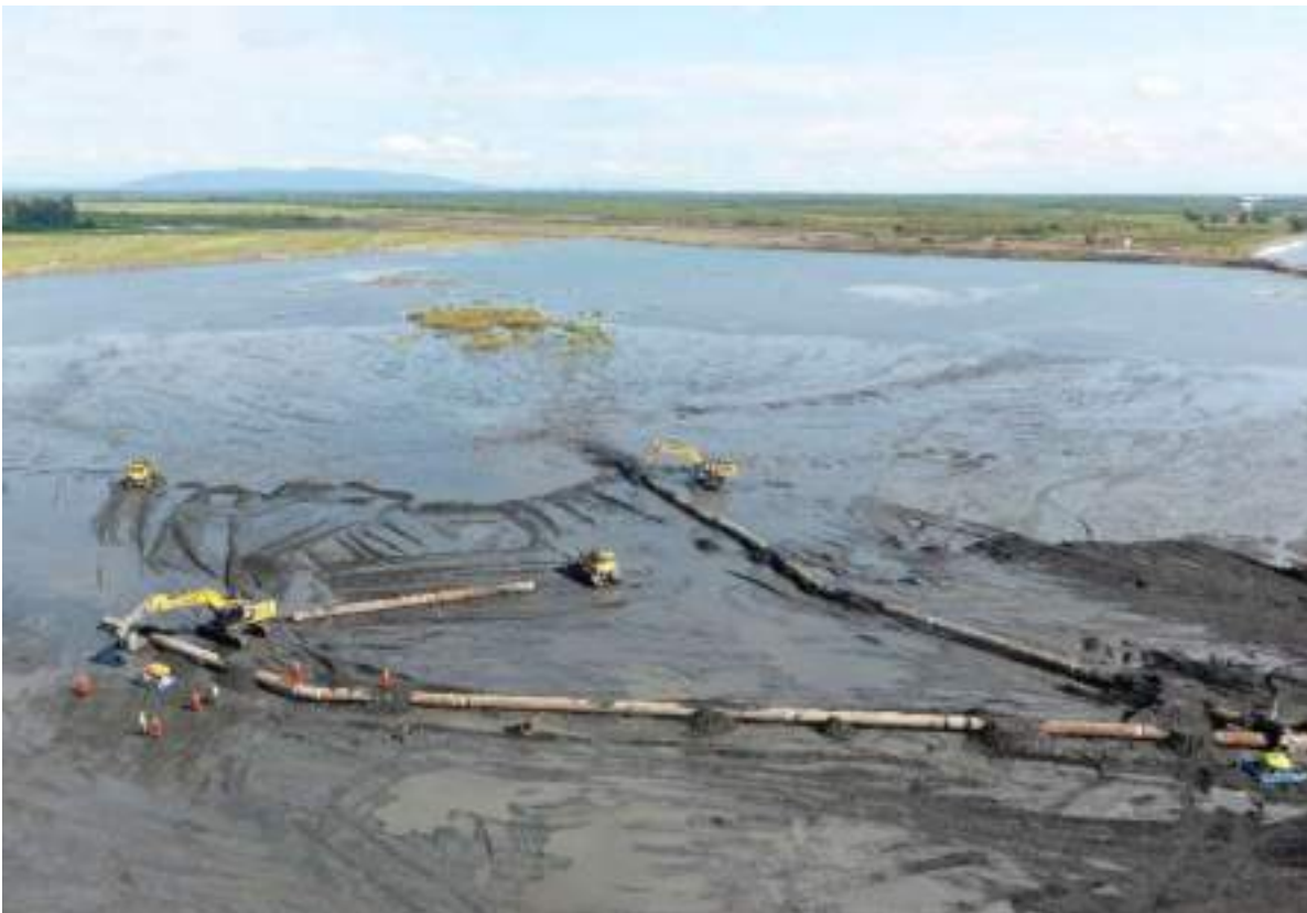
Figure 9-3 Splitting of shore pipeline to different areas
