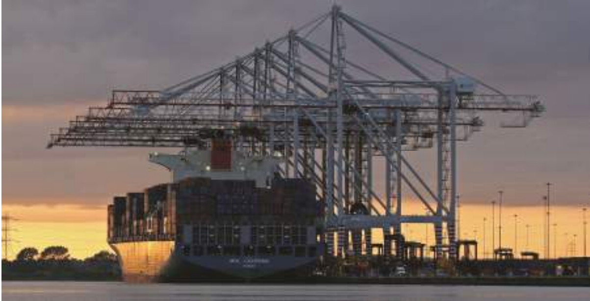
Figure 7-4 Typical RMQCs Operating at Berth
