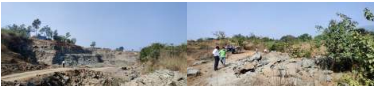
Figure 8-21 Kirat Quarry Location
