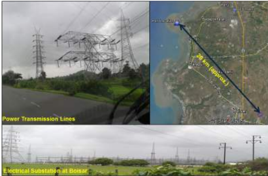
Figure 2-10 Location of Boisar Substation
