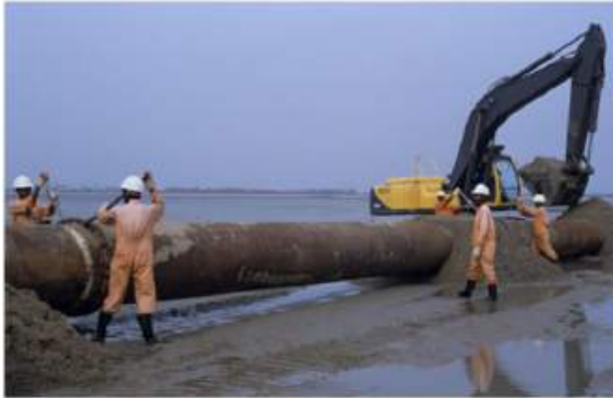
Figure 9-4 Extension of pipeline at reclamation area
