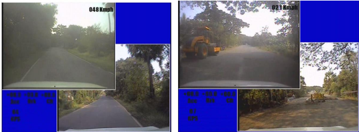
Figure 3.3 Narrow roads and diversions in road section of MSH 4
