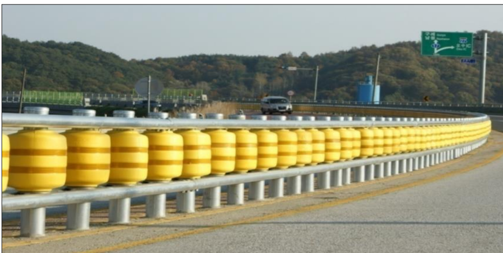
Figure 4-18 Rolling Crash Barrier
