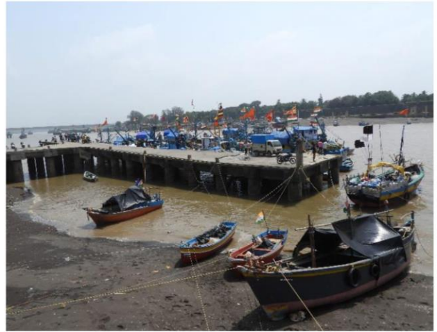
Boat Jetty Site, Daman Port
