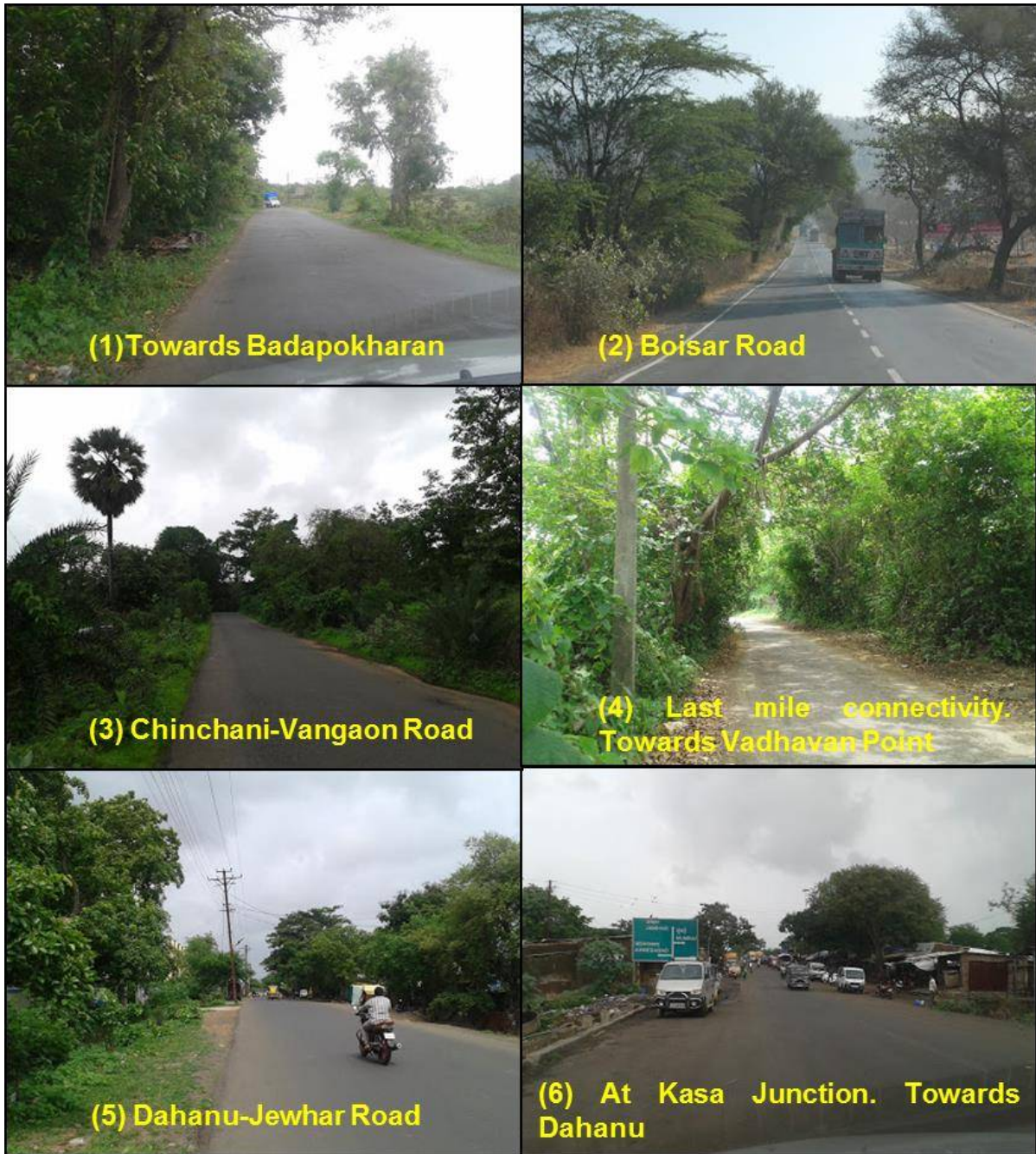
Figure 2.23 Road connecting to Vadhavan Port Site
